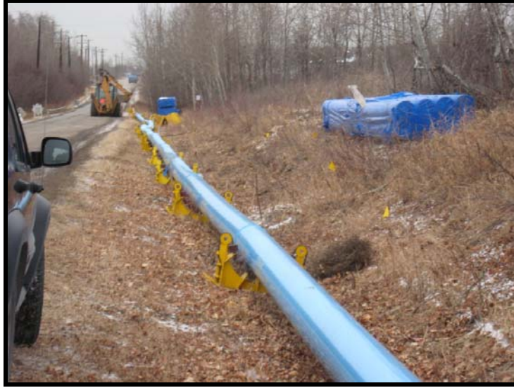
Figure 5. Rollers Used for Pullback Operations
