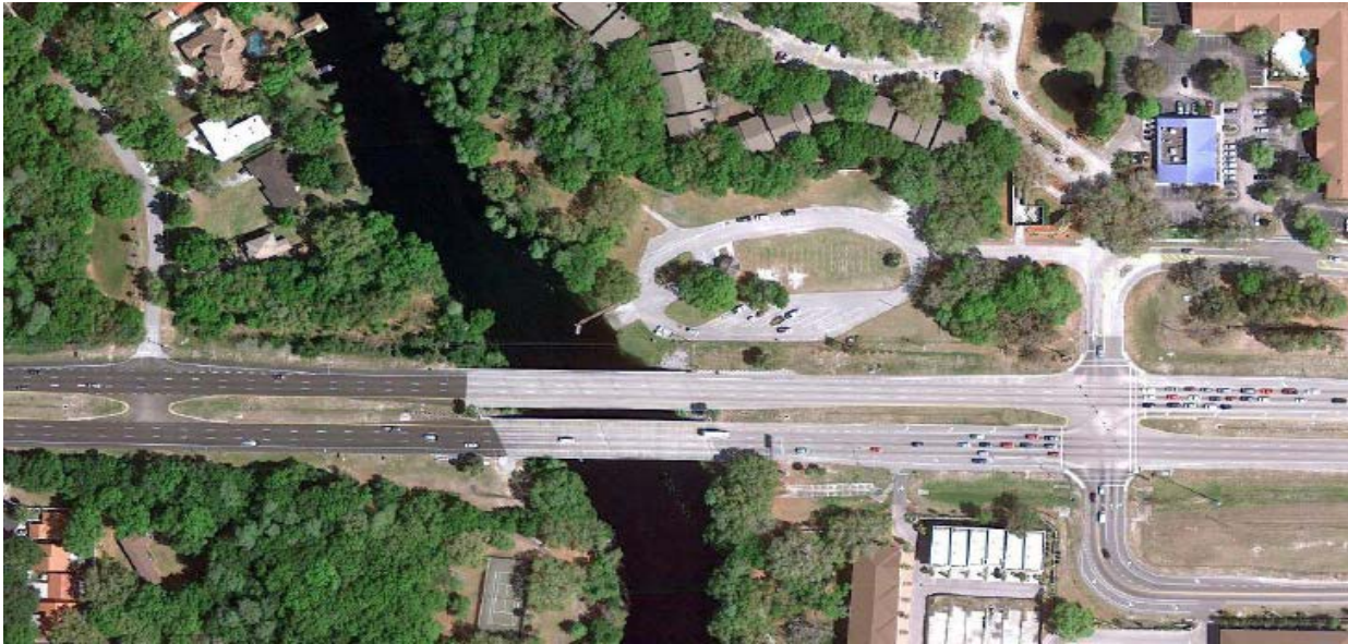
Figure 1 - Fowler Avenue crossing the Hillsborough River - Looking North
