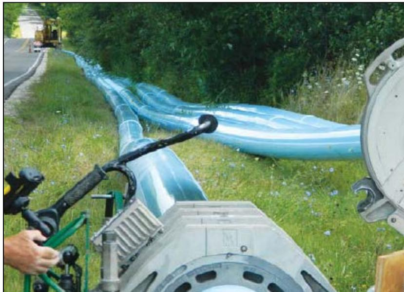
Figure 7. Pipe fusion and layout alongside roadway
