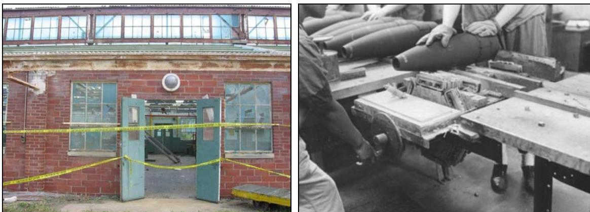
Figure 2. Manufacturing plant where laborers made ammunition during World War II [outside view (left); workers using stenciling machine to show correct zone and lot numbers on shells (right)].
