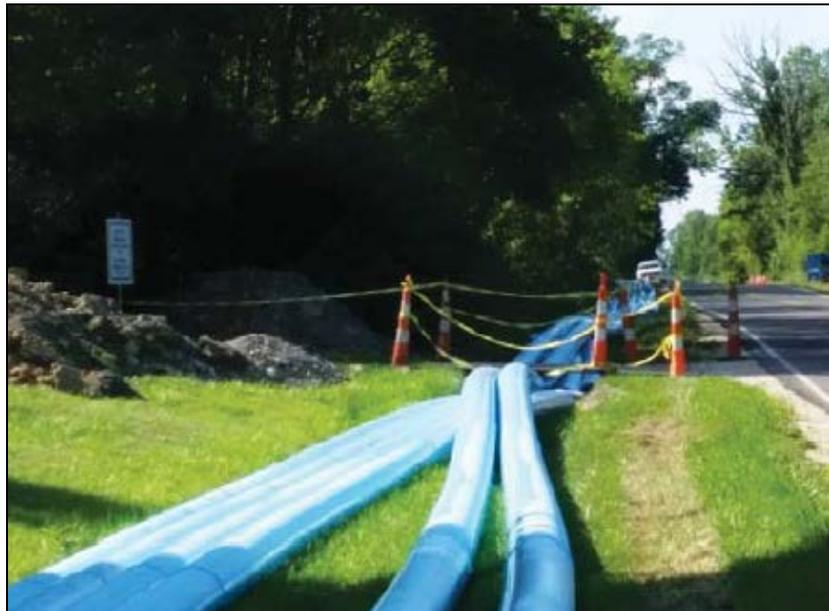
Figure 9. FPVCP staged along the side of the road ready for installation
