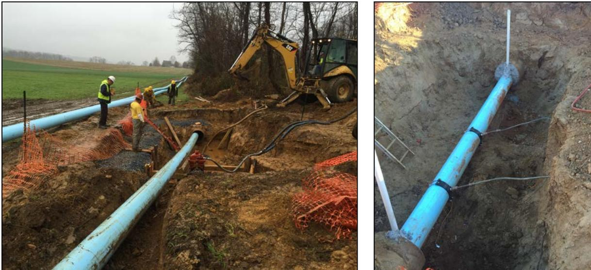
Figure 4. Pipe Installation [12-inch FPVCP water main entering 24-inch cast iron main (left); grouting of annular space with vent tubes and service connections (right)]
