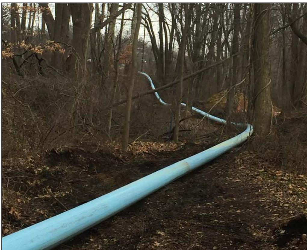
Figure 5. Pipe string staged along through trees, ready for pull-in
