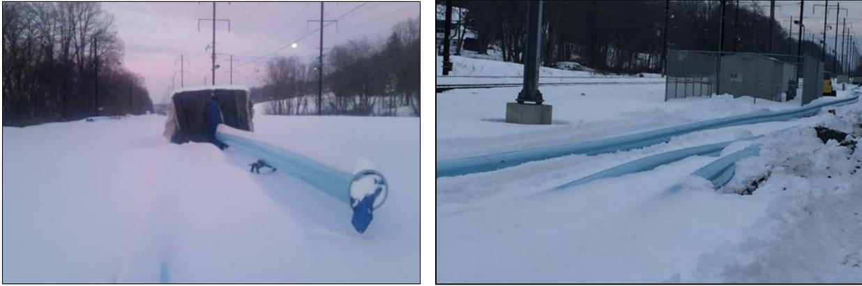
Figure 6. Pipe fusion during the cold weather season (machine setup (left); pipe layout after snow storm (right))
