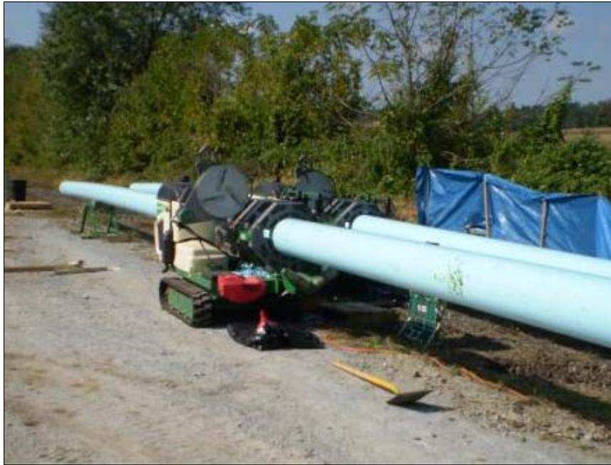
Figure 7. Fusion machines side by side
