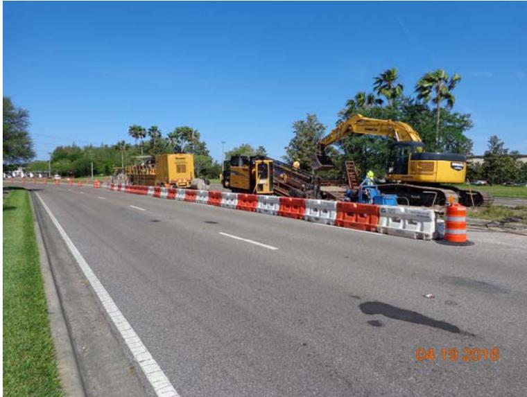
Figure 4: Mobilization of drill rig and supporting equipment within the median of Citrus Park Drive
