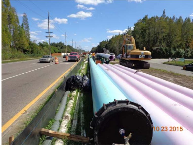
Figure 7: Pipe fusion and low pressure leak testing within Gunn Highway median.
