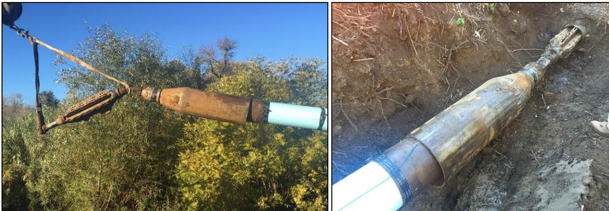
Figure 9. Installation from entrance pit [cutter and expander assembly (left); initial pull into existing steel (right)].
