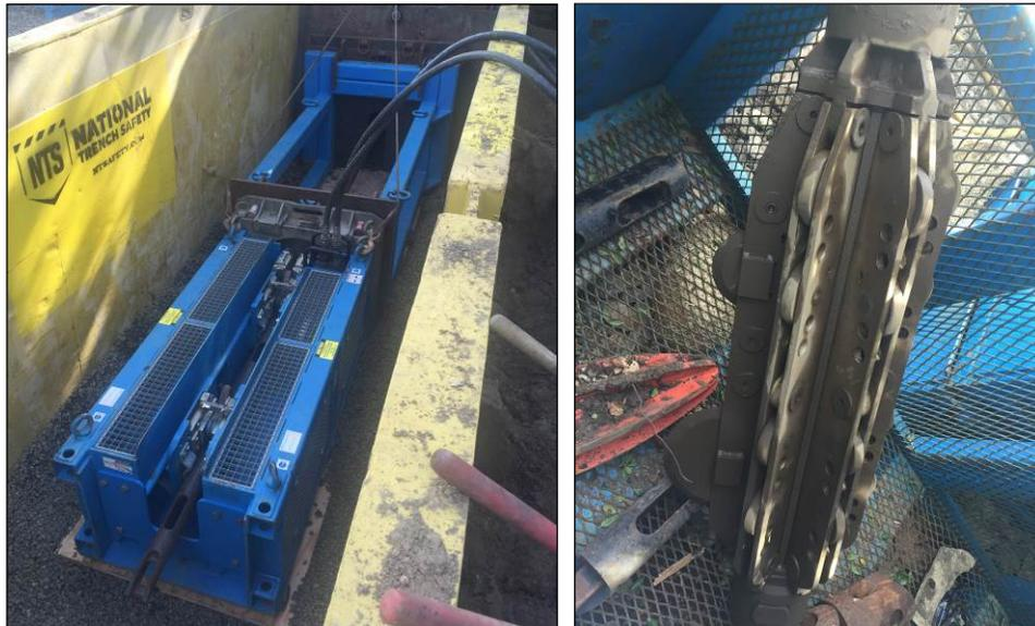
Figure 8. Static pipe burst equipment [static pipe burst unit in exit pit (left); roller cutters (right)].
