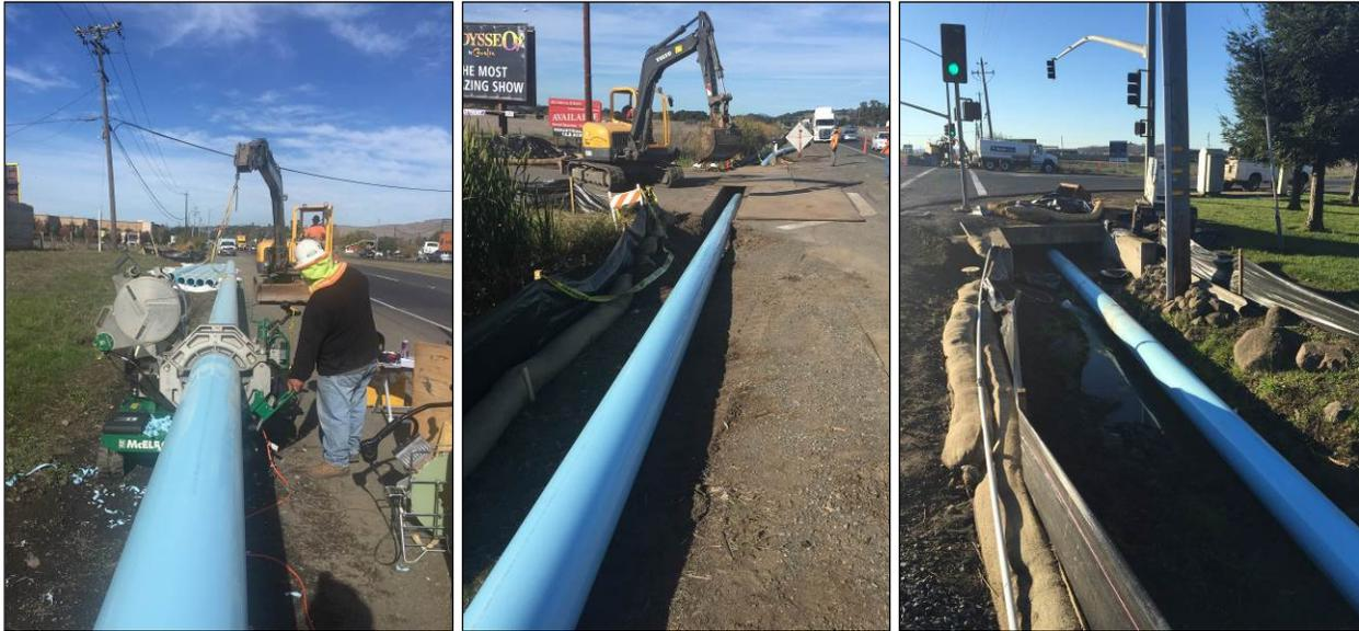
Figure 7. Pipe fusion and layout [fusion (left); layout under road (center); layout through culvert (right)].
