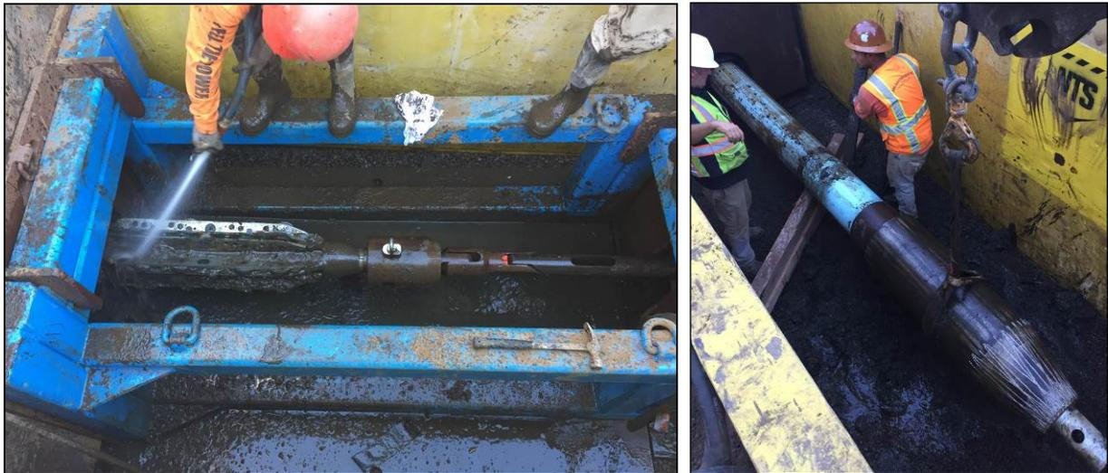
Figure 10. Installation from exit pit [roller cutter pulled through (left); pipe pulled completely through (right)].
