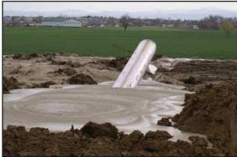
BTrenchless crews pull the 24-in.-diameter C-905 pipe back through the horizontally-drilled hole in the trenchless installation performed along Sheridan Boulevard during summer 2007.
