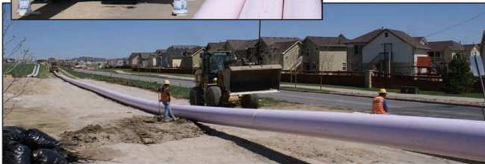
Broomfield is extending its distribution pipeline for non-potable irrigation water to correspond with expansion of the wastewater reclamation facility that will increase treatment capacity. The City and County is utilizing new technology developed by Underground Solutions Inc. that allows C-905 pipe sections to be fused together, eliminating joints and the need for joint restraints. BTrenchless, a division of BT Construction, performed the HDD installation this summer.
