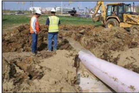
BTrenchless crews pull the 24-in.-diameter C-905 pipe back through the horizontally-drilled hole in the trenchless installation performed along Sheridan Boulevard during summer 2007.
