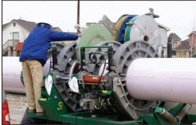
Fusible PVC™ from Underground Solutions has distinctive properties that allow for full-strength butt fusion joints under a patented process.
