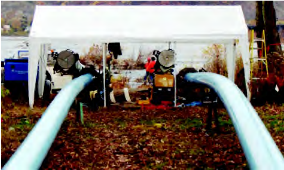
Figure 2: Two fusion machines were used to increase production.
