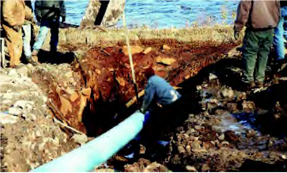
Figure 4: 12-inch product being inserted into a 16-inch iron main.
