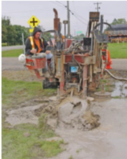
A Ditch Witch JT2720 is used on the directional drilled portion of the Riga Township water main project.
