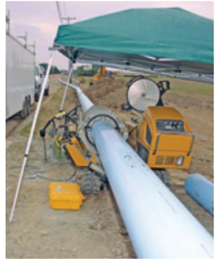
12-inch C-900 polyvinyl chloride water main is fused together for the Riga Township project.
