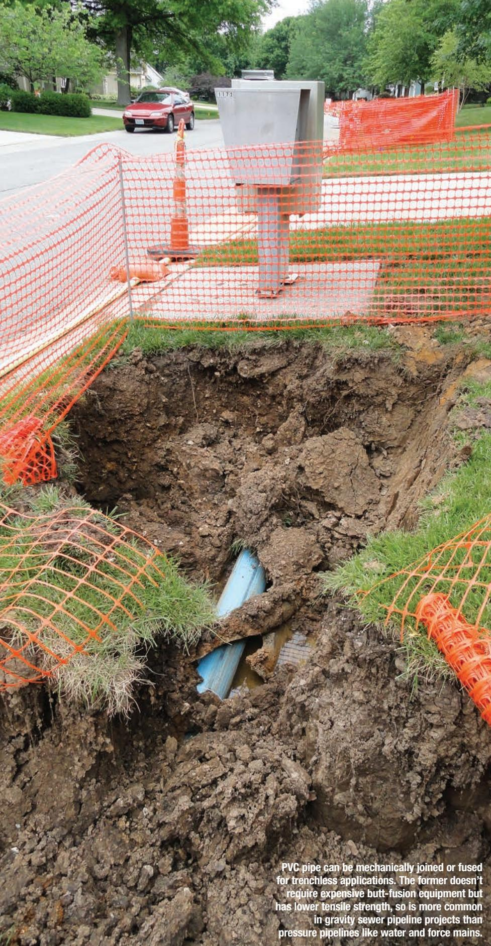
PVC pipe can be mechanically joined or fused for trenchless applications. The former doesn't require expensive butt-fusion equipment but has lower tensile strength, so is more common in gravity sewer pipeline projects than pressure pipelines like water and force mains.
