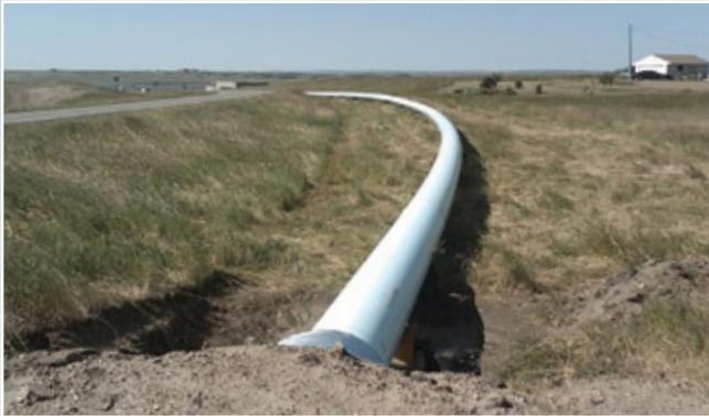
Installing temporary culverts allowed the entire length of PVC pipe to be fused together in a single string.
