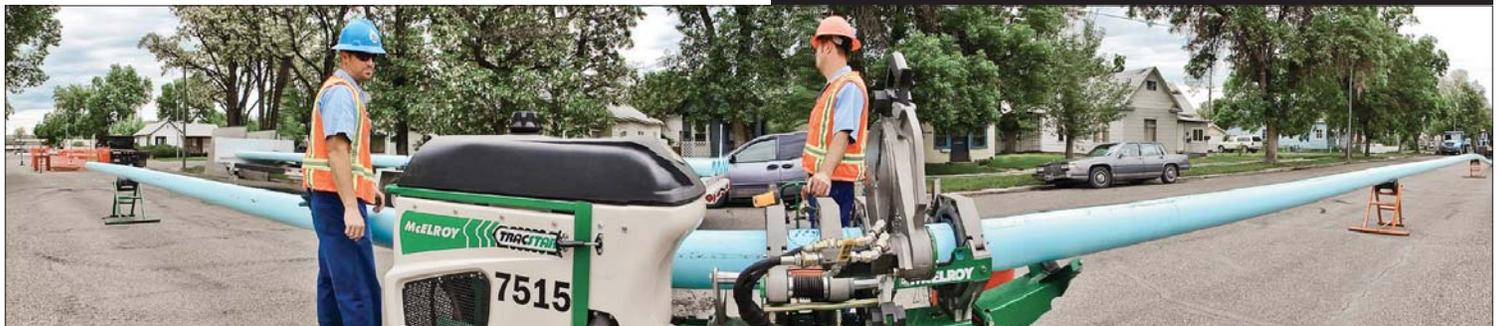
nect the new pipe to the existing line. Lustig says it takes about an hour and a half to burst and pull the new pipe through a 400-foot section. “We generally do one block at a time,” he says.
