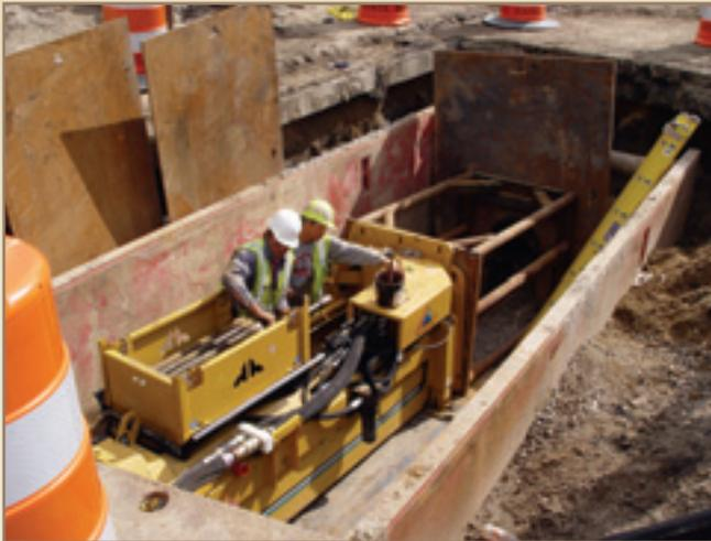
A Vermeer HammerHead HB 125, 125-ton static pipe bursting machine installs Underground Solution Inc.'s polyvinyl chloride pipe on the project.
