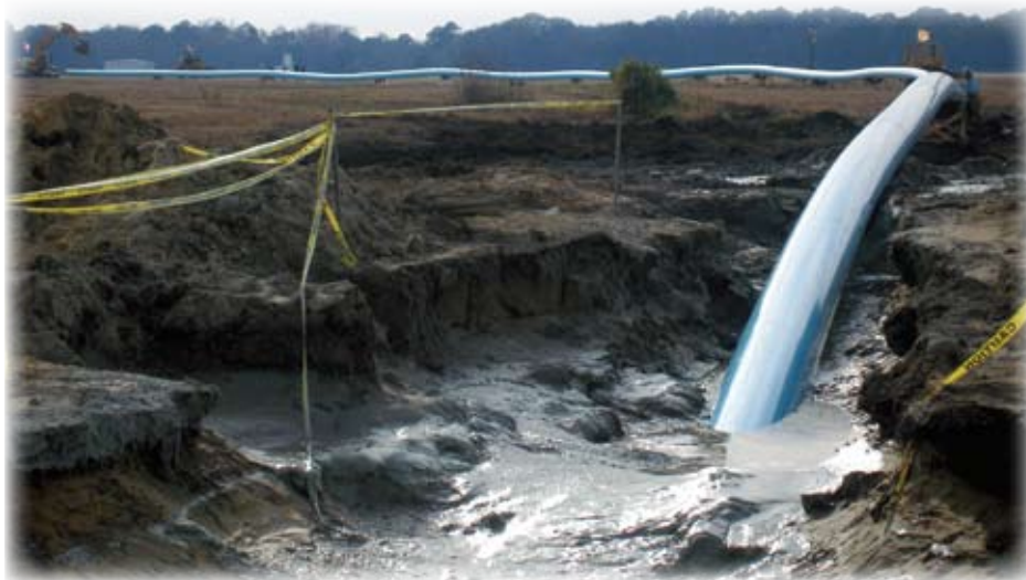
Pull-in began at 8:00 a.m. on February 15 and was completed 14 hours later.
