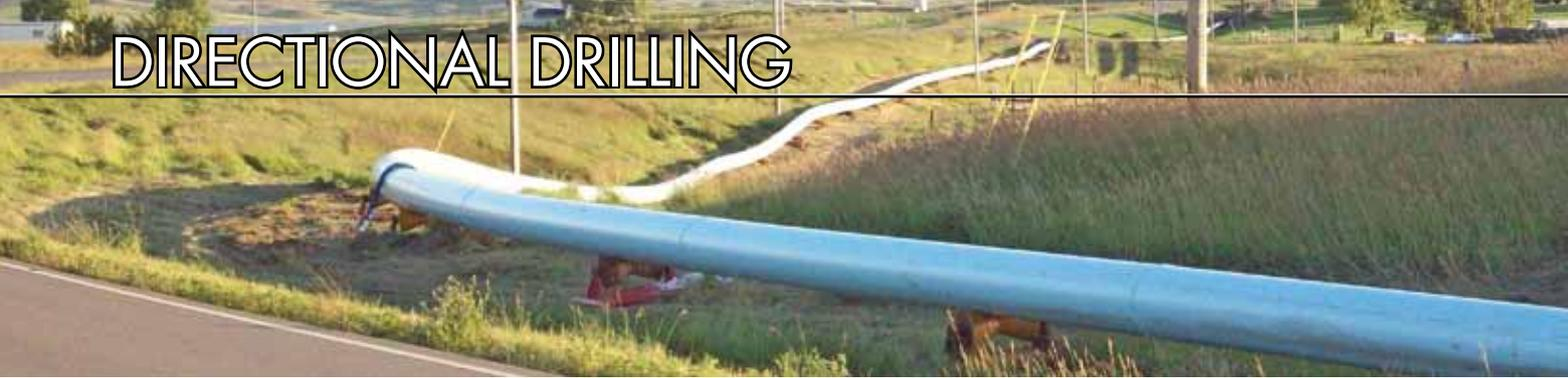
The fusible PVC pipe was snaked around the highways and driveways, waiting to be pulled into the ground.
