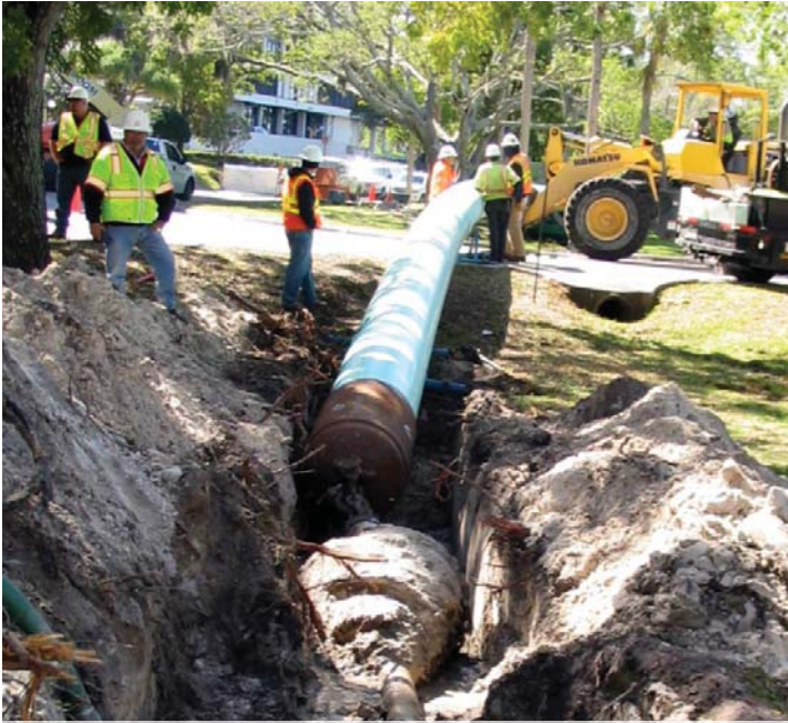
Horizontal Directional Drill
