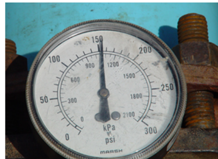
The taps were pressure tested to 150 psi for a period of one hour with no leakage. Both the dry and wet taps were successfully pressure tested.
