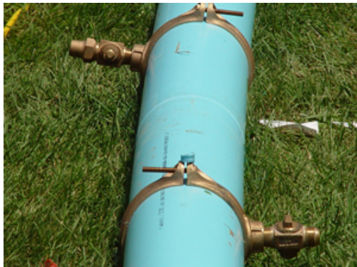
Taps were performed and corporation stops were installed at 12 o'clock, 9 o'clock, and 3 o'clock orientations. They were also located about 18 inches from fused joints.
